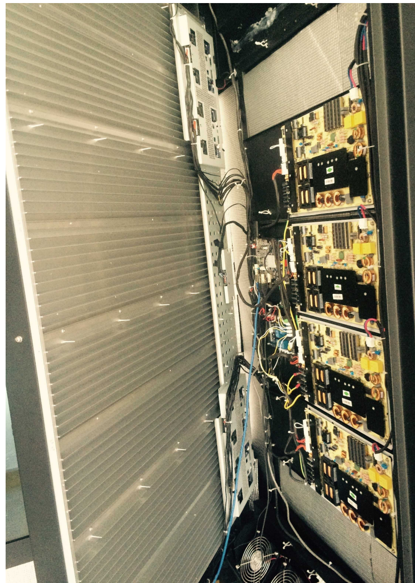
Air cooled fan system is key with heat disbursement
